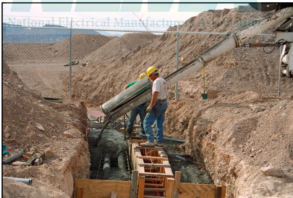
Example of Concrete Encasement
