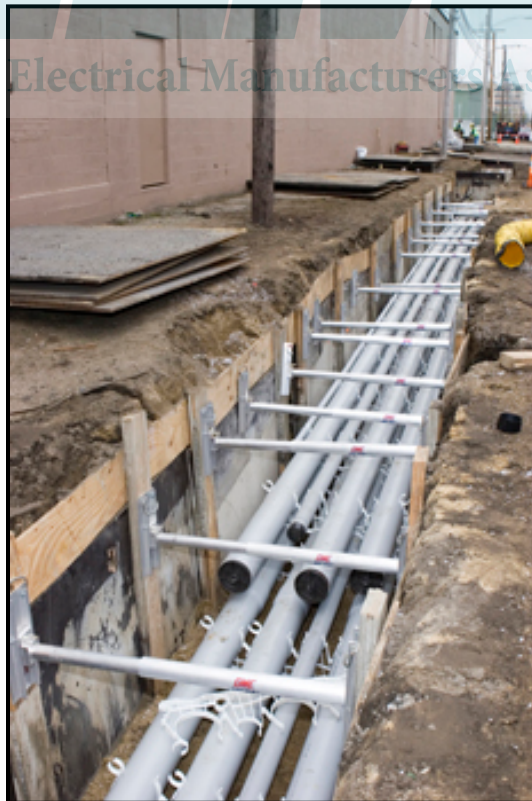
Routing of Raceway in Trench
