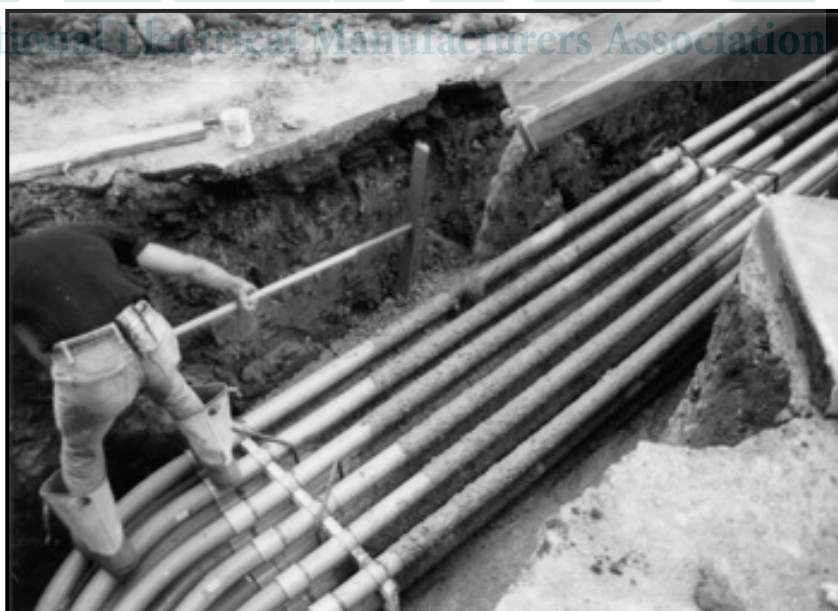
Backfilling of Trench
