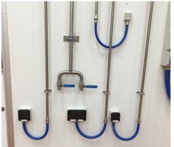
"It was critical that the cable protection system specified not only met the appropriate food industry hygiene standards but could also withstand the rigours of frequent wash down routines, where connections will be subject to extended wet and/or damp conditions.
