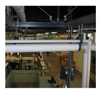
Use AICKINSTRUT for excessively wet or corrosive applications, including: refineries, chemical plants, pulp and paper facilities, aquariums, theme parks, cooling towers, and underground vaults.
